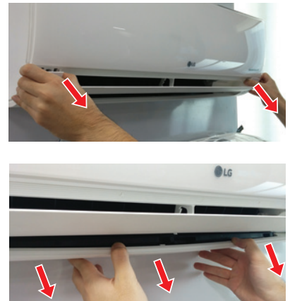
Figure 42: Removing the Bottom Cover, Alternate View.
