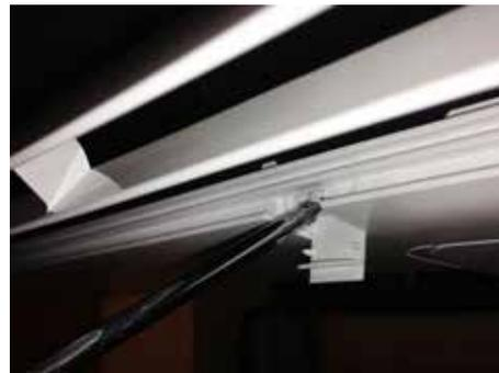
Figure 66: Remove (and Reattachment) Bottom Panel
