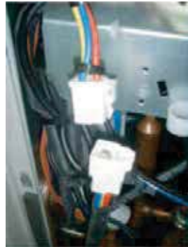
Figure 50: ARUN060GSS4 and ARUB060GSS4 Error No. 29 Compressor Terminal and Wiring Connections.
