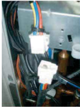
Figure 48: ARUN060GSS4 and ARUB060GSS4 Error No. 22 Compressor Terminal and Wiring Connections.
