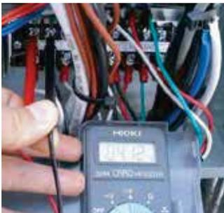
If the DC voltage between communication terminal A, B of indoor unit fluctuates within -9V ~ +9V, then the communication from the outdoor unit is normal.
