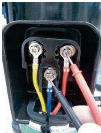
Compressor wiring connections.
