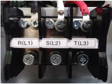
\* Compressor wire connector connection
