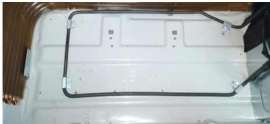
Figure 40: Drain Pan Heater.
