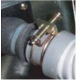
Clamp the Flexible Drain Hose Connection
