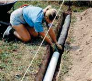
Figure 76: Underground Refrigerant Piping.
