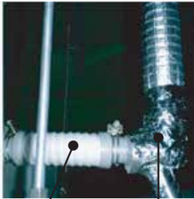
Figure 53: Properly Insulated Condensate Drain Piping.
