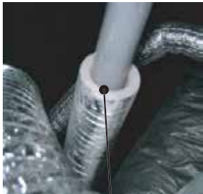
Figure 53: Properly Insulated Condensate Drain Piping.
