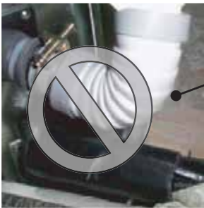
Figure 54: Condensate Drain Piping Should Not Include Sharp Bends.
