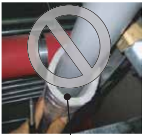
Insulation that does not fit—too loose
