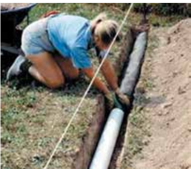
Figure 259: Underground Refrigerant Piping.
