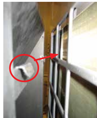
Figure 28: Close up of Wind Baffle Hangers and Where to Attach Them.
