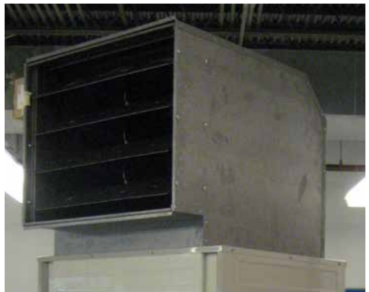
Figure 15: Installed Top Discharge Elbow.
