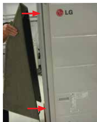
Figure 19: Positioning the Side Wind Baffle.
